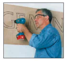
3. Mark holes with center punch, then drill 1/4" holes 3" deep where indicated on your template. Remove the template and clean out all drill holes using any of
